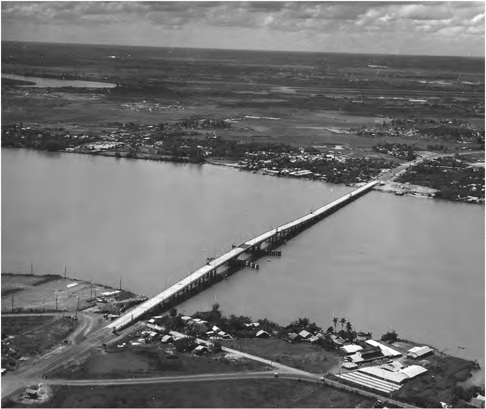
Bien Hoa Bridge, completed in 1972 by RMK-BRJ, was part of a new bypass road north of Saigon.
